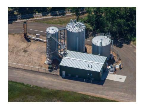
When Burnette Foods' existing Biological Aerobic System became difficult to operate due to overloading conditions, they decided to add an Anaerobic Pretreatment System ahead of it to provide a smoother operation and allow for additional future production capacity. The core technology for this upgrade project was a High Rate Anaerobic Granular Sludge Bed system, UASB.
